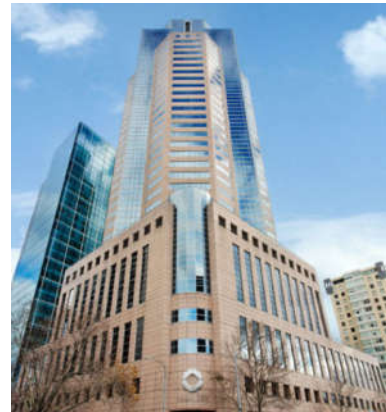
2 Lonsdale St Melbourne VIC Completed date: 2020 Application: Façade Windows Product: Prestige PR40 Area: 3,432 m 2
